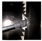
Make a 3/4" slit in the pleated filter where the gap in the vent cover is. This part of the vent cover should be facing away from the roof peak and down slope. Insert fan unit plug end through the slit from inside out, feeding the rest of cord out and placing fan unit up inside vent cover opening. This is now considered a complete powered fan unit.
