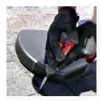
Using the provided gasketed self-tapping screws secure the vent cover and fan unit assembly to the roof deck and dab some sealant on the secured screw heads for added seal protection. Fan power cord should be extended out of the housing with about 20" of length available.
