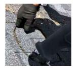
Using a reciprocating saw, cut along each line from one hole to the other until the piece is about to be fully cut. Use your free hand to grab one corner then finish the cut and discard the cut piece.
