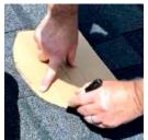
Use the cardboard template to mark a space centered between the roof rafters (trusses) of your desired location. Use a permanent marker to outline the template well as sawdust will make it difficult to see during the cutting operation.
