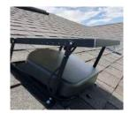
Connect the power cord on the solar panel to the fan unit and secure the power cord to the back leg of the solar panel mounting bracket using the provided zip tie and cut the excess off. Installation is now complete.
