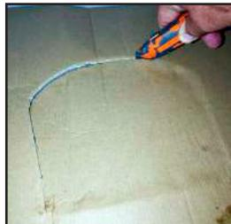
Make an impression using the piece of cardboard in the solar attic fan box. Cut out impression 1-2" outside the creased lines. The cutout will be your hole cut template for the roof.
