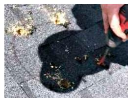
Drill a 1" hole in each corner of the outlined shape through the roof deck.
