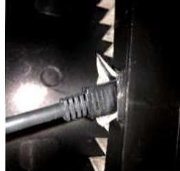
Pull out bottom of pleated filter where the gap in the vent cover is. This part of the vent cover should be facing away from the roof peak and down slope. Insert fan unit plug end through opening from inside out, feeding the rest of cord out and placing fan unit up inside vent cover opening. This is now considered a complete powered fan unit.
