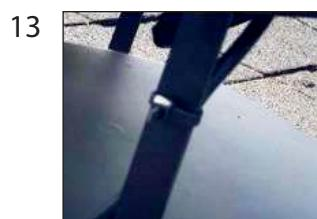
Connect the power cord on the solar panel to the fan unit and secure the power cord to the inside of the riser bracket using the provided zip tie and cut the excess off. Installation is now complete.
