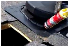
Once this is complete, apply a  $\frac{1}{4}$ " –  $\frac{1}{2}$ " bead of roof sealant around opening under the shingles and around the top of the vent cover.
