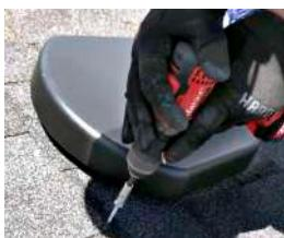
Using the provided gasketed 2.5" self-tapping screws secure the vent cover and fan unit assembly to the roof deck and dab some sealant on the secured screw heads for added seal protection. Fan power cord should be extended out of the housing with about 20" of length available.
