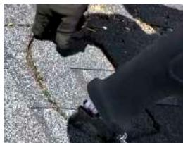
Using a reciprocating saw, cut along each line from one hole to the other until the piece is about to be fully cut. Use your free hand to grab one corner then finish the cut and discard the cut piece.
