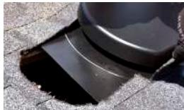
Gently slide vent and fan unit up under the shingles until the vent housing is about  $\frac{1}{2}$ " from the top of the hole cut. Secure any other loose shingles around vent cover using some sealant.
