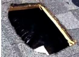
Using a prybar, gently pry up shingles out to 5" around the cut opening removing any nails that you come in contact with that could obstruct installation of the vent and fan unit. Test fit the vent cover and fan unit.
