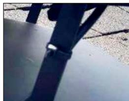
Connect the power cord on the solar panel to the fan unit and secure the power cord to the inside of the riser bracket using the provided zip tie and cut the excess off. Installation is now complete.
