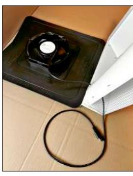
Cut a 8-9" square or circle in sidewall (gable or crawlspace). Fit fan unit in cut hole checking fitment. Feed fan plug and cord through back of anti-gust vent and down through the animal intrusion guard so all cable slack is outside of vent. Nestle fan into the back of the vent cover.
