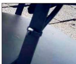
Connect the power cord on the solar panel to the fan unit and secure the power cord to the inside of the riser bracket using the provided zip tie and cut the excess off. Installation is now complete.
