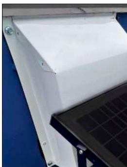
Dry fit fan and vent cover assembly into sidewall hole cut ensuring flush fitment. Cut away siding or anything that will prevent a tight seal against home.
