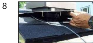
8 Ensure bottom flange seats in existing roof vent hole to check vent and fan fitment.
