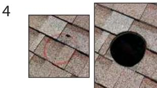
Existing Oversized Attic Vent or no existing Attic Vent: Mark and cut a new hole in Roof to size that corresponds to Fan circumference (approximately 7-8" in diameter) and follow instructions below.
