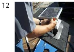
12 CAPTURE MAXIMUM SUN! After connecting the fan cable to the solar panel, adjust solar panel to approximately 10 degrees from horizontal towards the south or southwest if possible. \*
