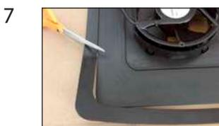
Carefully cut scored lines if necessary to fit & insert fan ensuring tight fit. Full size is for 75 sq. in. vents.
