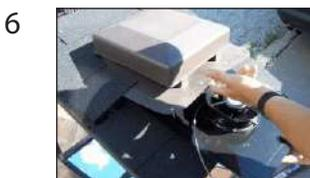
Lift up vent and insert fan and check for fit.
