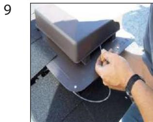
9 Feed fan cable through the vent near the bottom, up and out, (not between the vent and shingles) then replace the vent to its original location. If you have a vent with a screen, cut a 1/2" slit in the screen and feed the cable through the slit. Lift up or insert fan and vent together, apply a 1/2" bead of roof cement around circumference of hole, then return to its original location. Secure vent and fan to roof deck with (8) x 2" roofing screws uniformly around the cover perimeter.
