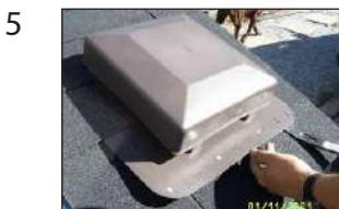
Existing attic Vent: Gently pry up shingles around vent, and existing vent using a flat bar. If vent has inside collar or can restrict airflow, replace with new vent. If not, follow instructions below.
