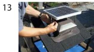
13 After securing the panel to its most efficient adjustment, Ty-rap the cable to the adjustment leg to secure the cable.
