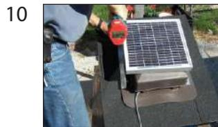
10 Mount solar panel to roof with 4 screws using the included sealing tape cut into 4 equal pieces at each screw location.
