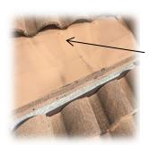
**4.** Existing Oversized Attic Vent Installation (No new penetration created). Locate two static vent hoods in separate locations of attic (if not possible then use a single vent as shown in step 8). Gently remove pest screening on vent from roof.
