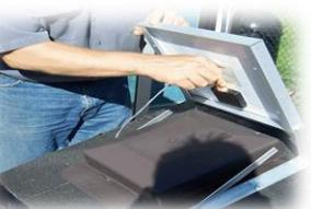
**6.** Feed fan power cord through opening of vent to outside by going over internal air dam and out. Fan should be positioned at a slight angle to ensure proper attic air exit.
