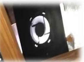
**5.** Fan Install: enter the attic and locate oversized attic vent. Use 3/4"-1" wood screws with washer to secure fan assembly to underpart of roof sheathing. (If sheathing is 1/2" or less do not fully seat screw)
