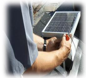
**10. Capturing Maximum Sun** - After connecting the fan cable to the solar panel, adjust solar panel to approximately 10 degrees from horizontal towards the south or southwest if possible. \*
