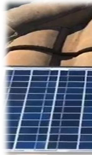
**9. Direct to Clay Tile Mount** - Mount the solar panel directly to clay tile by positioning panel rails in troughs of tiles, mark screw holes, and drill 1/4" diameter holes through clay tiles without going through sheathing then mount panel to roof using 4 provided screws with sealing tape ensuring adequate compression into sheathing.
