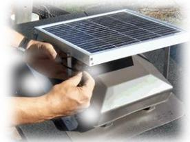
**11.** After securing the panel to its most efficient adjustment, Tie-wrap the cable to an adjustment leg to secure the cable.
